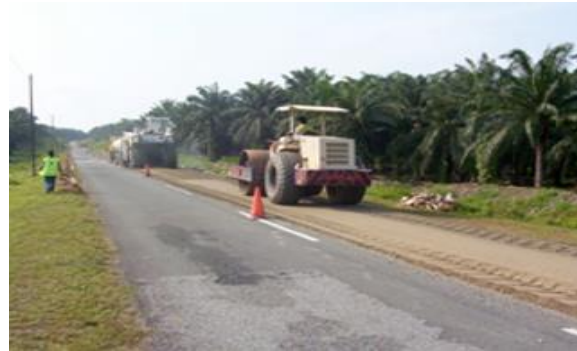
Figure 7. Process of initial compaction
