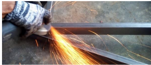
Figure 4 : Removing the rust
