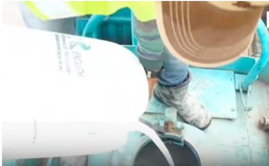
Figure 6. Polymer base is added and mixes into the water tank in the recycler machine
