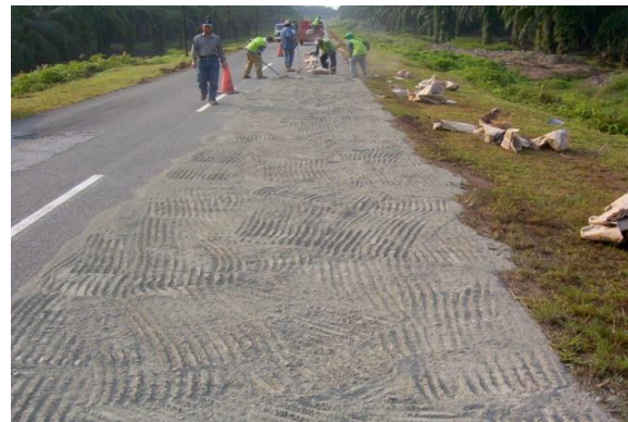
Figure 3. Spreading stabilizer using hand raker
